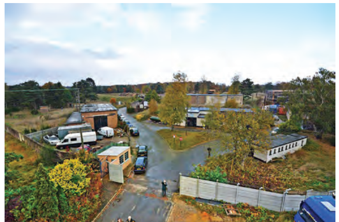
A cluster of buildings at the site entrance seen from the entrance watchtower projecting timber platform. The large brick building on the left was another inspection and repair workshop, but probably for non-explosive material given the absence of blast walls. Maintenance Building 58 is to the rear of a Component Servicing building in the centre of the photo, and a toilet block is to the right in the foreground
